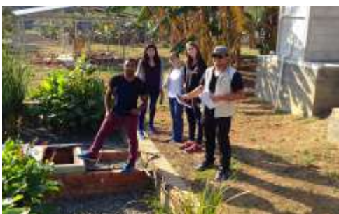
Students from the 2015 cohort (pictured from L to R: Mesai Loffe and Natalie Melgoza from CPP; Amy Bigelow, Heather Tegley, and Federick Pinongcos from SDSU) viewing the constructed wetland treatment system at the experimental field site run by the University of KwaZulu-Natal.
